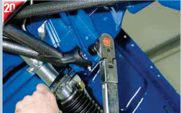
20 All fasteners are torqued to specifications at this time. Here, Richard torques the lower-control-arm pivot and steering-rack mount.
