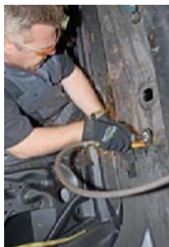
In the process, some seat clearance issues were addressed with the floor pan. A couple of slots were cut prior to bolting up the sub frame connectors.
