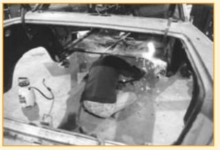
If a torch is used to cut the sheetmetal, be sure to have a water sprayer (visible under the wheel well) on hand to extinguish the flames that will probably result from the undercoating catching fire (water is much less messy than a fire extinguisher in this application).
