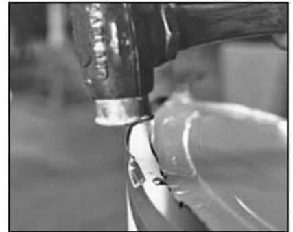
**14** A hammer is used to flatten the edge every few inches, joining the two sections. The rest of the protective plastic remains on the tub.
