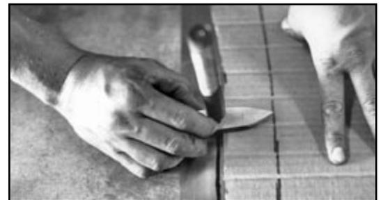
**15** Next, the cardboard assembly is removed from the car and slipped inside the wheel tub. Reversing direction of the contour tool (but using the same hole as before), Berg transfers the body contour from the cardboard onto the metal top section, as shown. Consequently, the black line on the left becomes the actual cut line for the metal tub.
