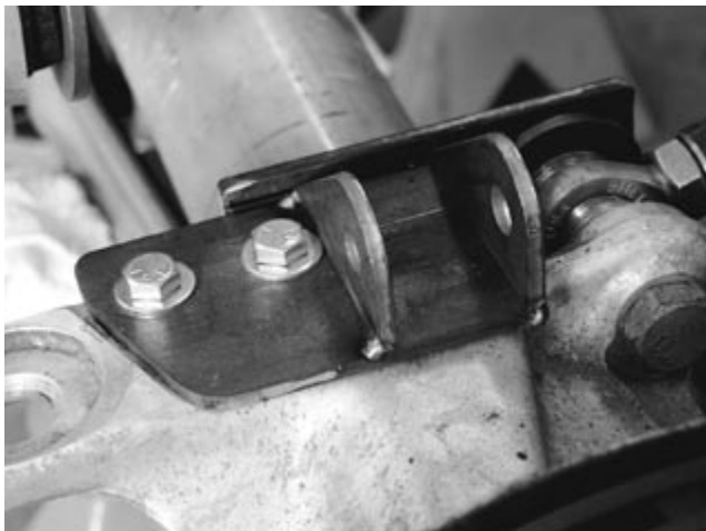
An additional piece of plate was added to the side of the bracket to add strength. It picks up the bolt that mounts the upper bar and will be welded to the main bracket after a little more trimming along the top. The brackets were tacked together for mockup and will be TIG welded completely once everything fits.
