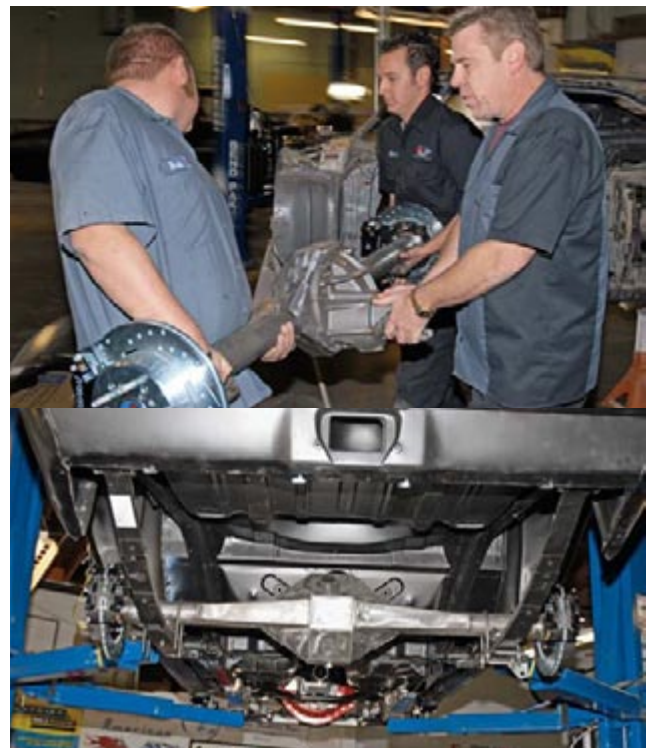
After the leaf springs are installed, the next step is getting the Currie "9+." rear axle housing in place. This is where having lots of friends is a good thing. And here's how it looks. In Part Four, we're going to install the fuel tank, exhaust system, and steering column. It's beginning to look like a car now.
