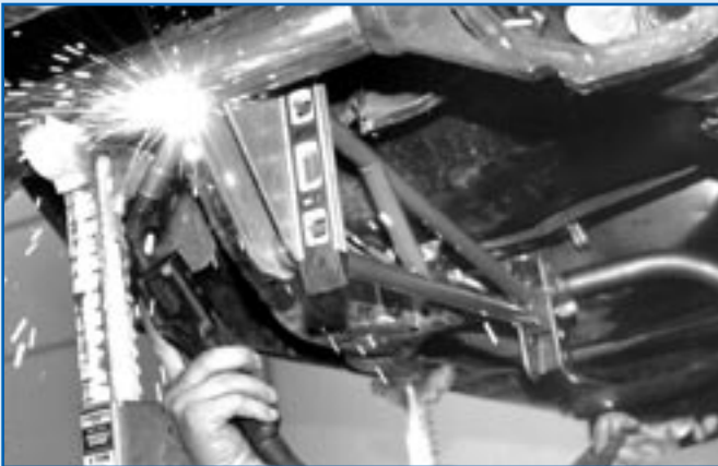
With clamps holding the front crossmember in place, the rear brackets are checked for plumb and tacked to the housing.
