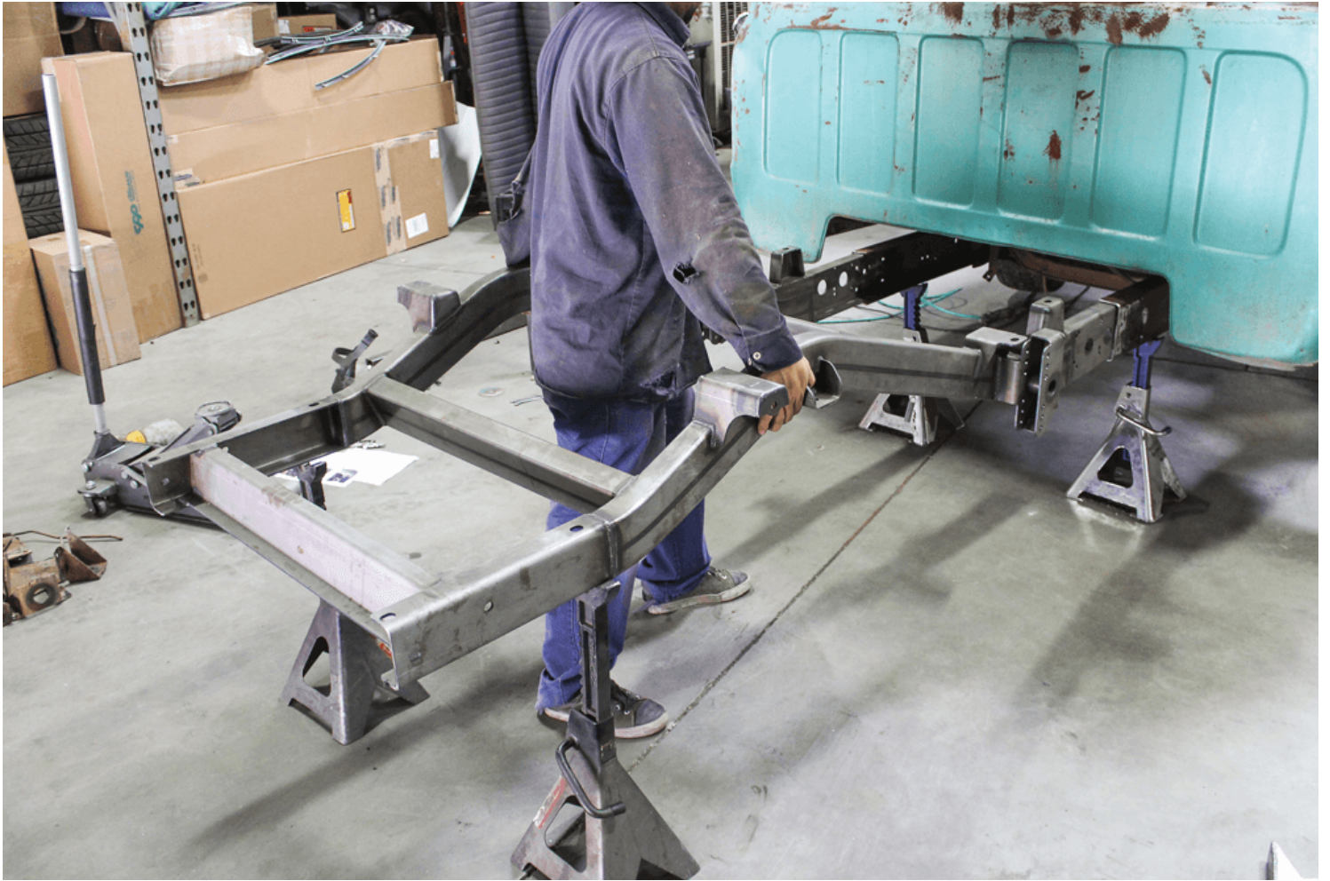
With jack stands in place, the new rear frame section was positioned and partially installed.
