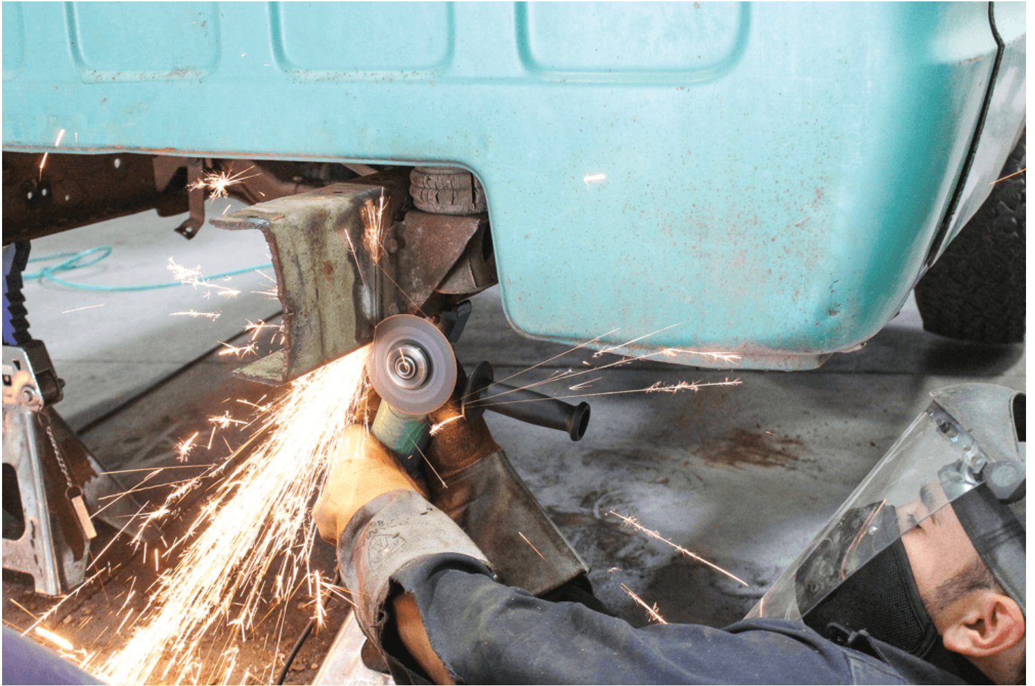
11 A combination of a sawzall and a cut-off wheel was used to make a perfectly straight cut down the frame rail.
