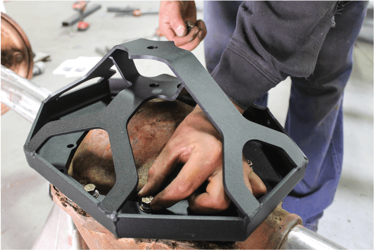
With the axle prepped, we installed the new Watts-link pivot bracket using the provided hardware.
