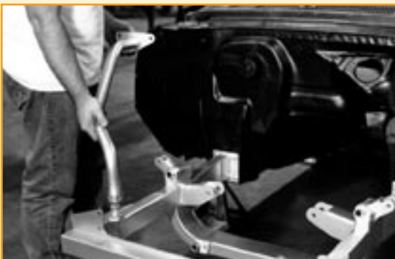
With the lower frame securely mounted, the front struts are installed. The tops of the struts attach to the firewall in the factory location.
